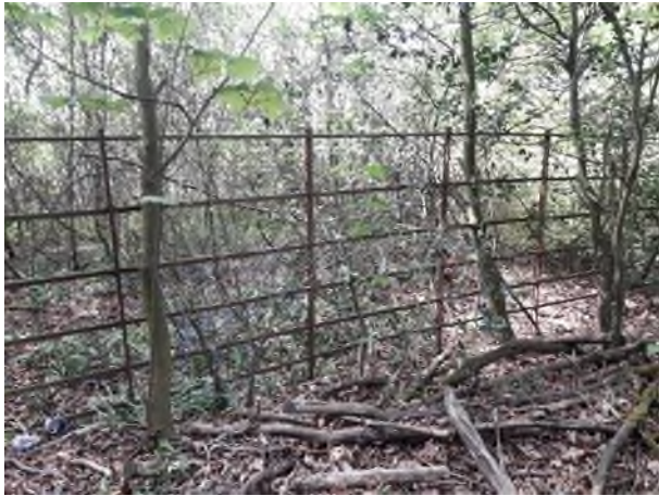
Intact metal railings
