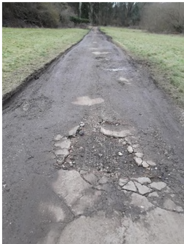
Surfacing of track along Footpath 02
