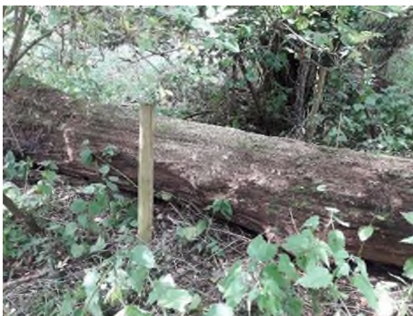
Fencing in The Dell damaged by a fallen tree
